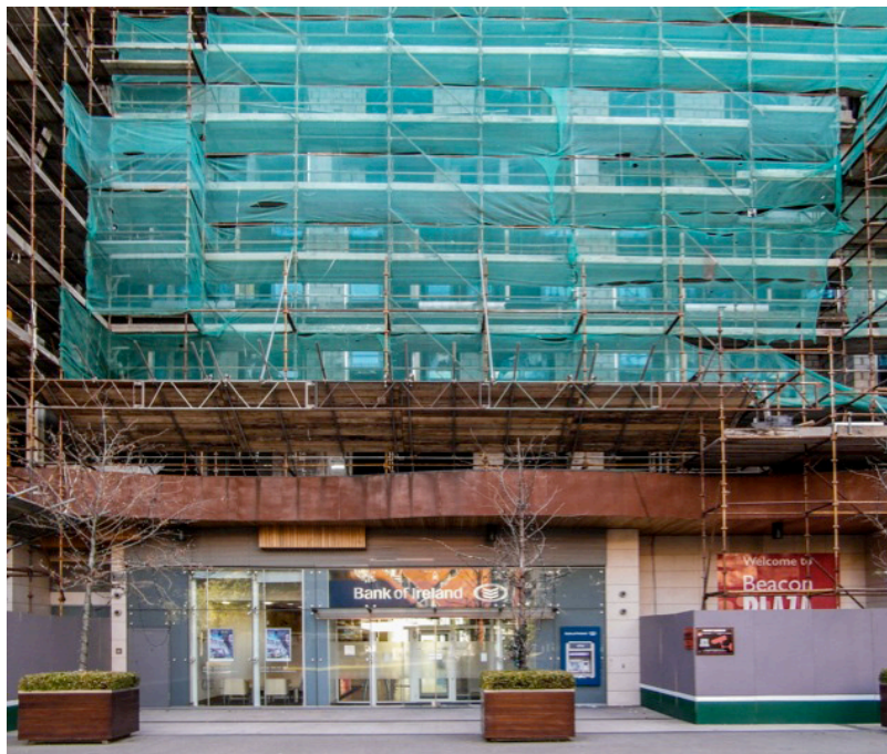
Figure 5: Example of ‘Carcass Occupancy,’ Beacon South , Sandymount, Dublin, Ireland. Credit: Lórin Vass.
